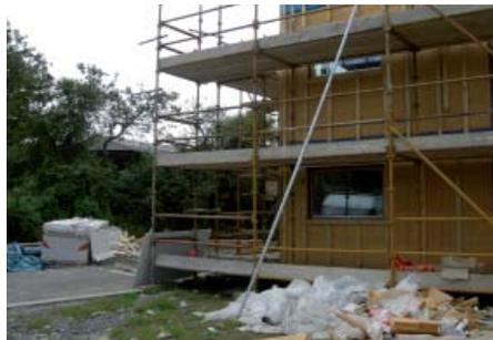
tion. The hemp-lime mix is applied directly to the medium-density fibreboard. The method is similar to what the Americans call Stucco. This cheap US-method consists of a simple timber frame clad with some type of external sheet and directly onto this the Stucco is applied without a ventilation cavity.
